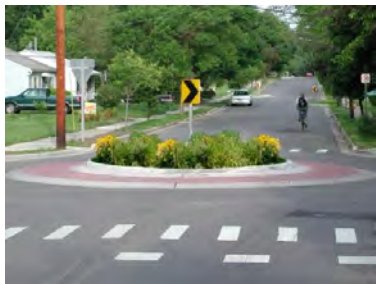
Traffic Calming Mini Traffic Circles help reduce speed at intersection without stopping
