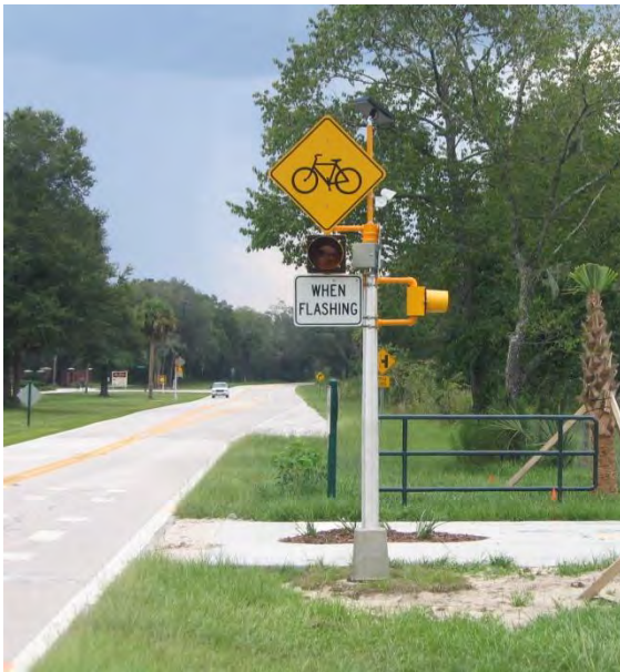
Fig. 9.7G. Active Crosswalk Warning Systems
