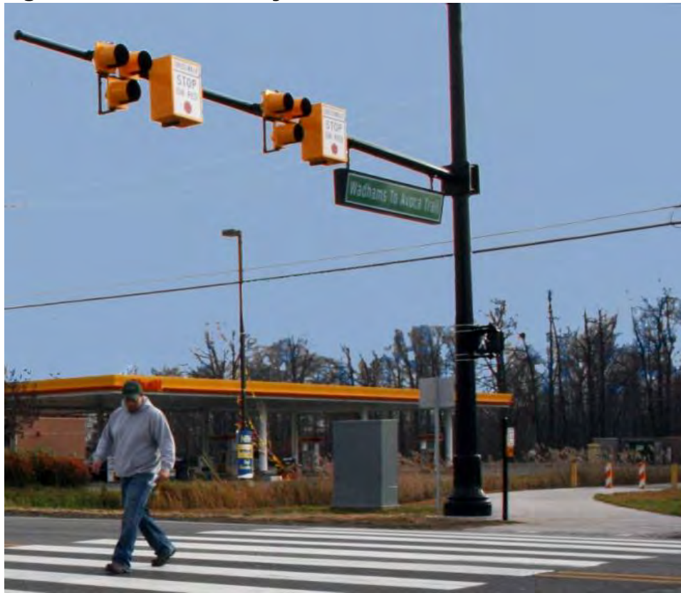
Fig. 9.71. Pedestrian Hybrid Beacon
